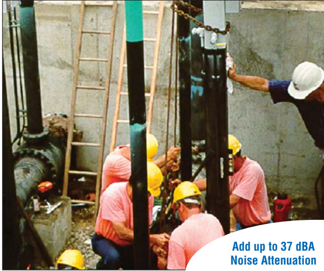
Figure 7 - Installation of Becker Below Ground Ball Valve Regulator.
