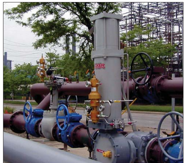
Figure 2 - Model FPCV-T0 Full Port Ball Valve provides guaranteed flow shutoff
